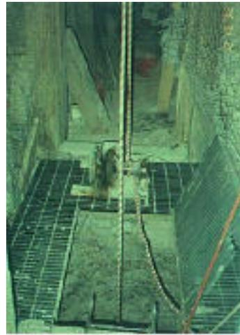
Bar grating with folding security hatch covering shaft and hoist
